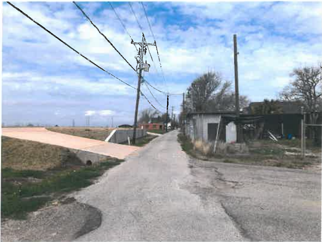
VIEW FACING WEST ALONG NORTH FRONT STREET
