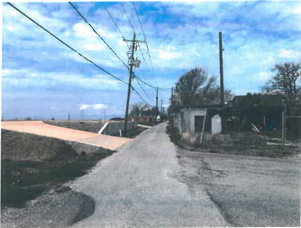
VIEW FACING WEST ALONG NORTH FRONT STREET
