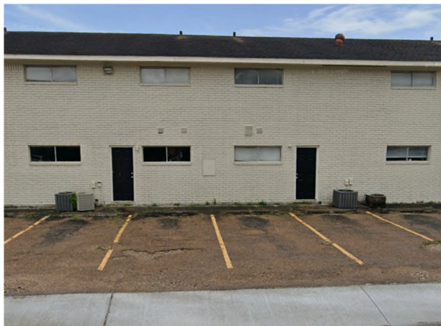
View of location of undeveloped alleyway from Arbutus Street, facing east
