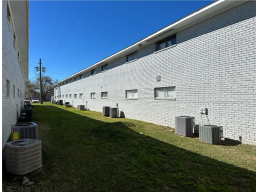
View of two of the three apartment buildings traversing the undeveloped alleyway
