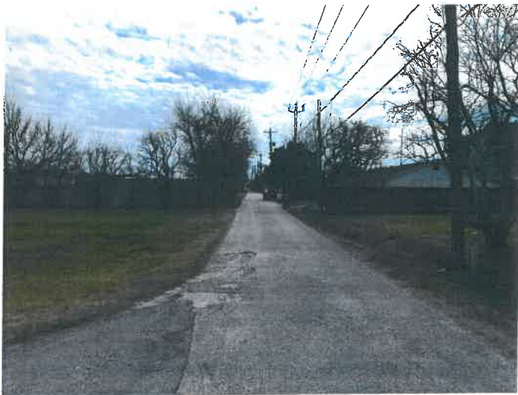
VIEW FACING EAST ALONG NORTH FRONT STREET
