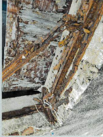
Deteriorated Walls & Window Frames
