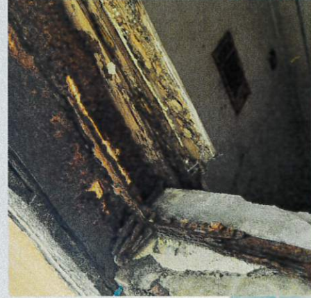
Deteriorated Walls & Window Frames
