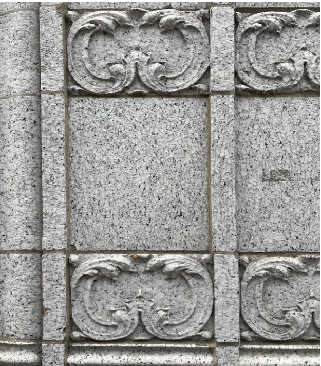
Figure 2d: Terra cotta gained popularity in the late 19th century as a cheap and lightweight alternative to stone. Glazing techniques allowed the blocks to imitate a variety of natural stone materials. Photo: John Sandor, NPS.
