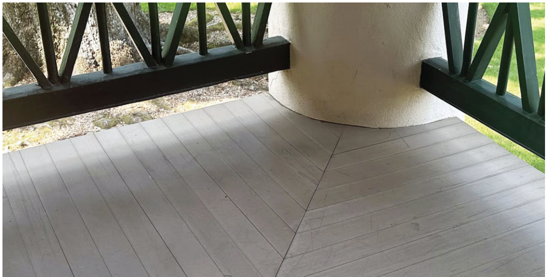
Figure 15. Tongue-and-groove porch flooring is manufactured in several different substitute materials. Each type has different properties, though most are more moisture-resistant than wood. The prefinished product shown can be painted when worn, but repainting is not recommended for some product choices. Photo: Oak Alley Foundation.
