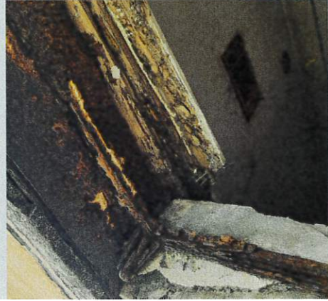
Deteriorated Walls & Window Frames
