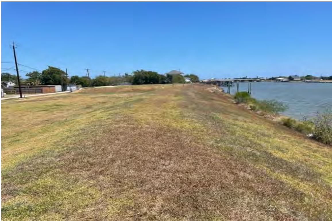
Alternate View of Subject Property
